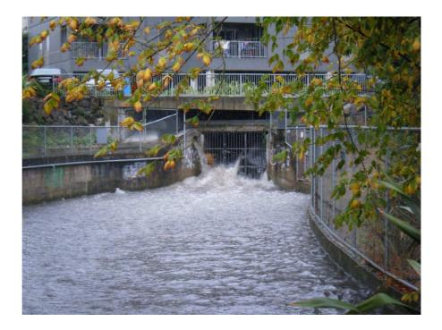
Photo of the Lyon Avenue CSO discharging a mixture of untreated diluted wastewater and stormwater (Note apartments directly above it)
